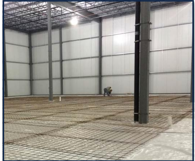
Shown covered with vapor barrier and metal mesh.
